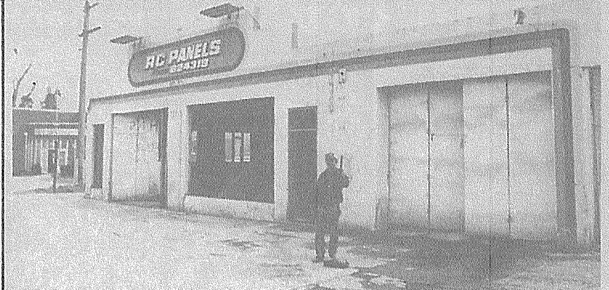
★ Ray Donkin working on the former service station.
