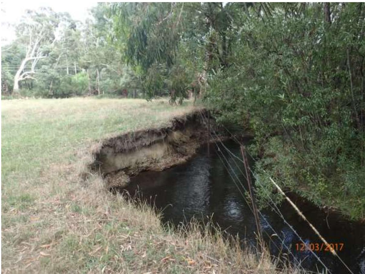
Photo in the Subject Area (Little Yarra River) showing the practical problems of fencing close to a meandering and migrating river within a floodplain.
